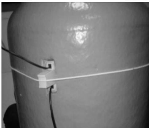
For a daisy chain installation of pipe/ tank sensors, it is important that you do not disturb the slider button positions, otherwise none of the pipe/tank sensors will communicate.
